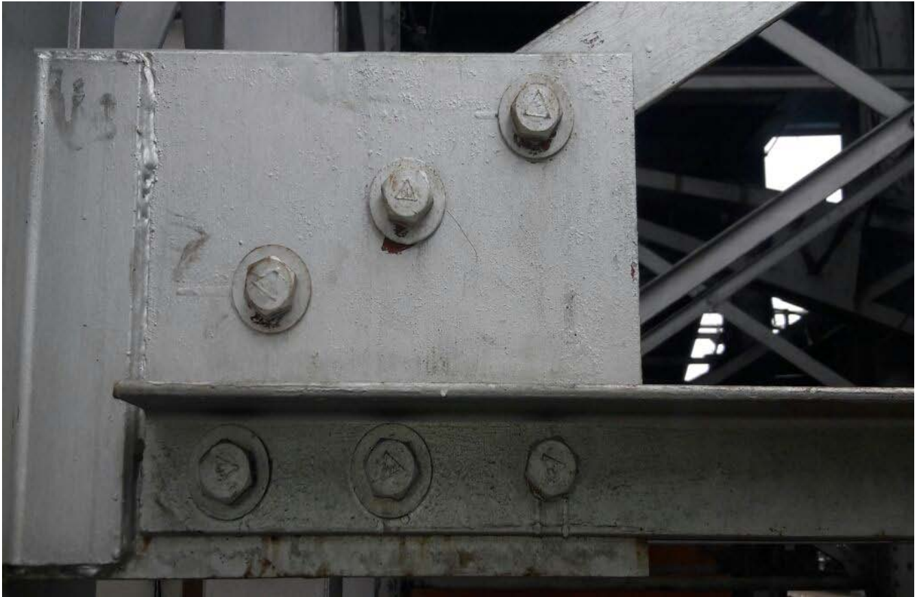
Angle Connected to Gusset plate by Bolted Connections
